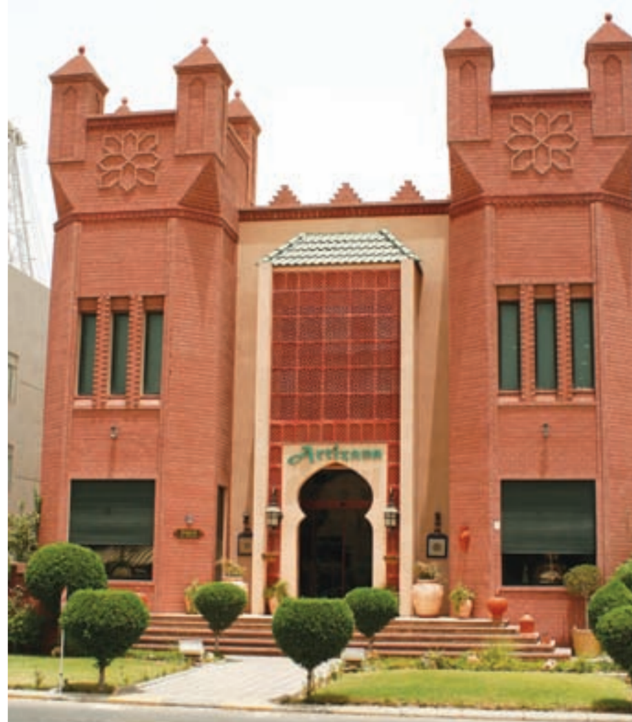
A store front view of Artizana, a home furnishing business in Free Trade Zone.
